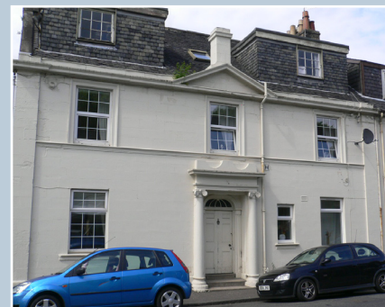
Badly designed box dormers detract from the classical proportions and elegant detailing of this late 18th-century house.
