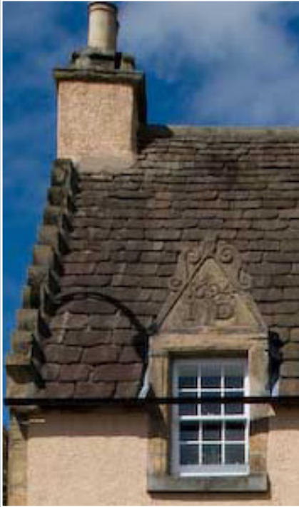
Graded stone slates, laid in diminishing courses from the bottom to the top of the roof. Associated features include crowstepped gables, a corniced chimney and a decorative dormerhead dated 1694. Elgin, Moray. © N. Haynes.
