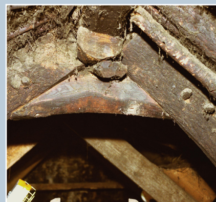
Hand-hewn roofing timbers pegged together in a late 18th- to early 19th-century cottage. Pitlochry, Perth & Kinross.
